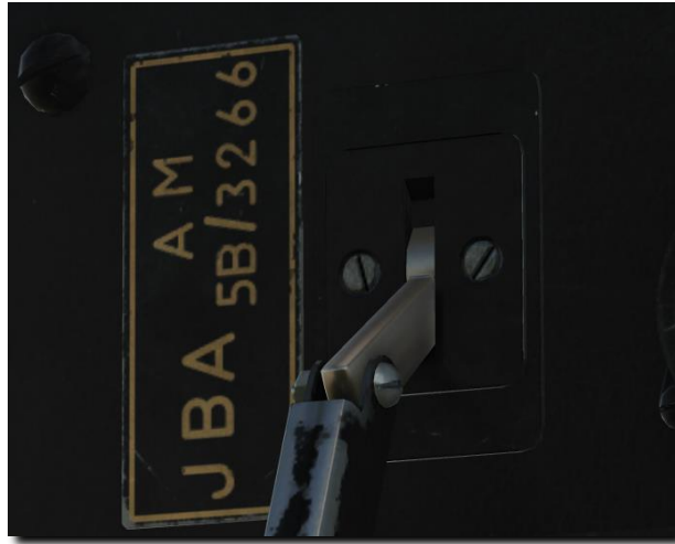
Figure 36: Electrical Services Switch.
