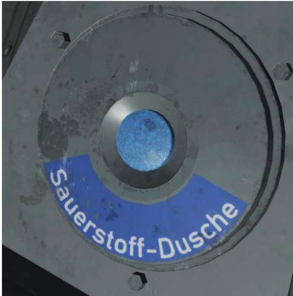
Figure 58: Emergency oxygen button
